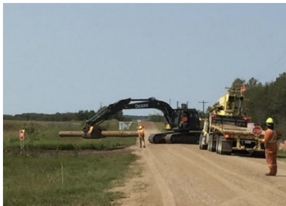
Excavator loading pipe – km 13+100 – Aug 1, 2018
