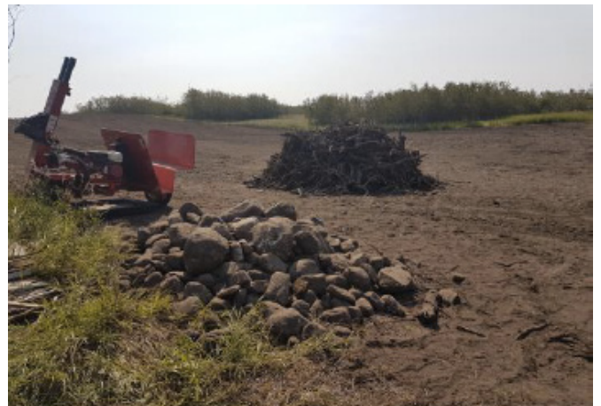
Rock and wood debris for disposal – km 6+490 – Aug 2, 2018
