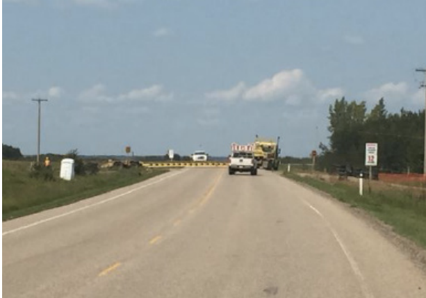
Excavator delivered to ROW – km 17+600 – Aug 2, 2018
