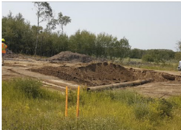
Exposed pipe – km 16+250 – Aug 2, 2018
