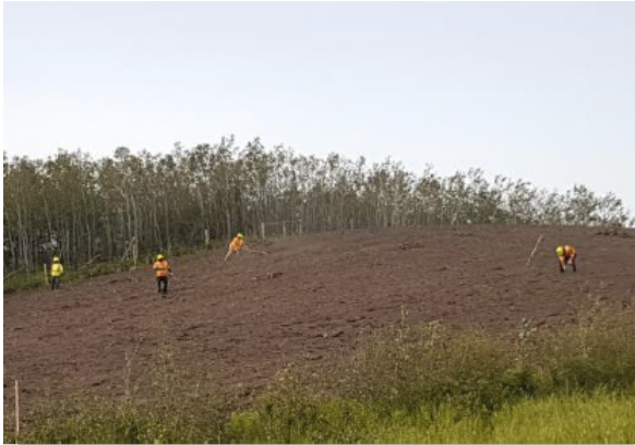
Clean up crew picking up debris – km 6+700 – Aug 1, 2018
