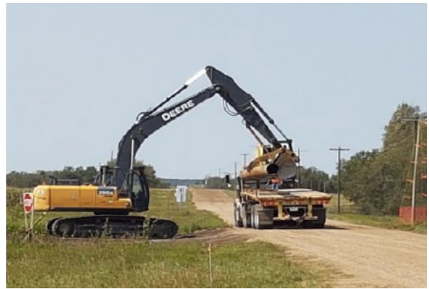
Excavator loading pipe – km 13+000 – Aug 1, 2018
