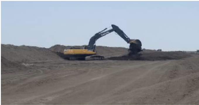
Excavator bailing and levelling out subsoil – km 121+900 – Aug 1, 2018
