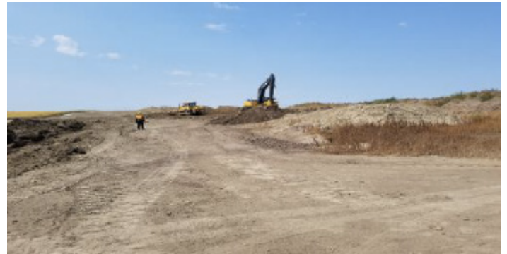
Levelling subsoil – km 127+450 – Aug 1, 2018
