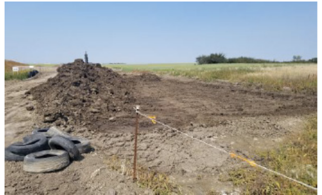
Excavator bailing out soil – km 118+000 – Aug 2, 2018
