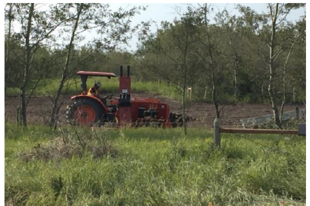
Tractor loading debris – km 6+500 – Aug 1, 2018
