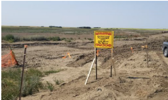
Signs are fixed and are more visible – SF 78 – Aug 2, 2018
