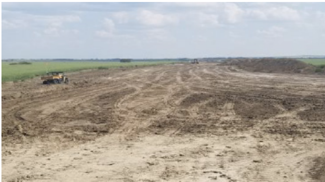
Grader levelling ROW – km 122+300 – Aug 3, 2018
