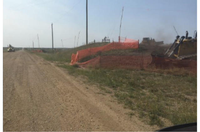
Snow fence down – km 8+300 – Aug 2, 2018
